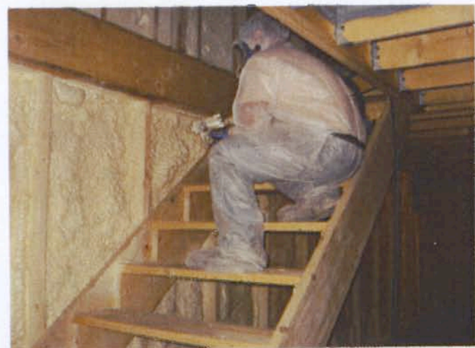
Sealing in the Heat. The crew hit the concrete substrate in the home's basement with 2 inches (5.1 cm) of E:zero's E:2000 closed-cell foam.
